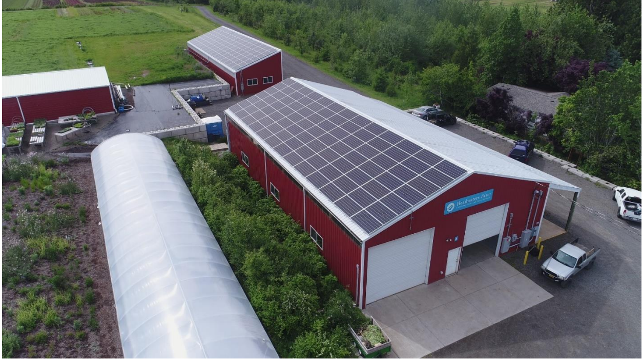
The 70.56kW photovoltaic system at Headwaters Farm is on two south-facing roofs with no seasonal shading.
