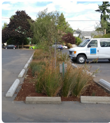
Left: Depave volunteers remove pavement from parking lot. Right: They replaced it with plants that filter pollutants out of rain as it runs off the lot.
